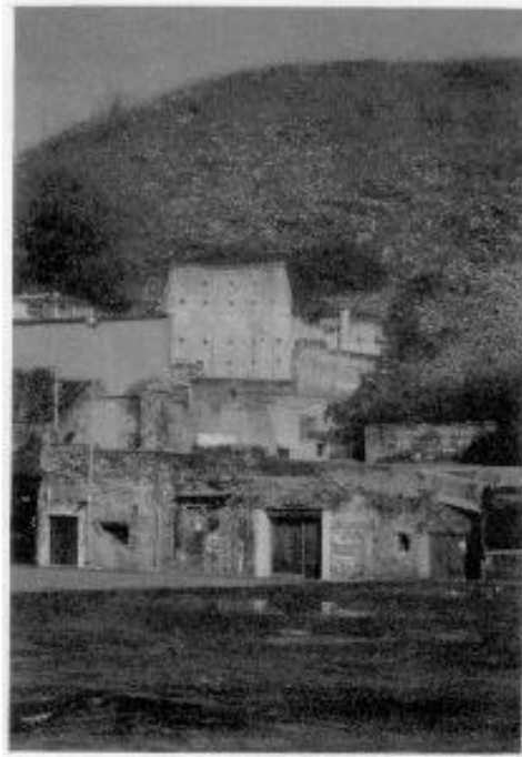
Plate 1. General view of the Monte Testaccio
